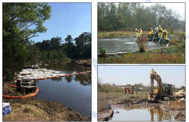
Figure 1: Spill response cleanup efforts may involve anchoring spill cleanup equipment like sorbent booms and skimmers on shorelines, agitation of river sediments, and physical cleaning or removal of oiled material by hand or with heavy machinery. Photos: Public Domain, courtesy of NOAA Office of Response and Restoration.<sup>6</sup>
